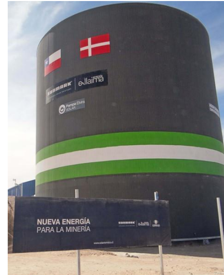
Picture from a project of F.W. Rørteknik of a 4'500 m 3 TTES in Chile
