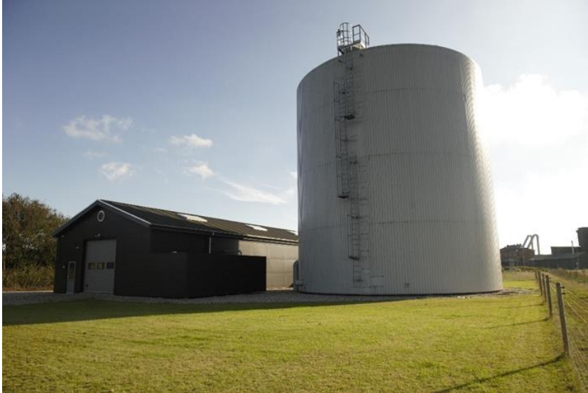
TTES in Karup (Denmark) – 3'600 m 3 . Photo: Karup district heating
