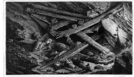
Fig. 84—Falling in of a 10m.
